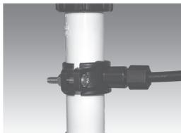
**Step B** – Slip drain tube through black compression nut. Insert drain tube into the opening in the drain saddle and hand tighten the black nut, and add 1/4 turn with a wrench.
