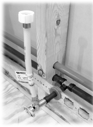
Flexible PVC riser, 1/4-turn crimp x compression stop, and PEX stubout bracket.
