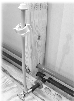
WaterPEX® riser, 1/4-turn CrimpRing™ x compression stop, and PEX stubout bracket.
