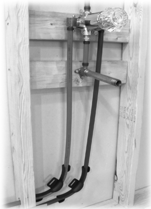
Rough-in at shower using adapters, elbows, drop ear elbow, and bend supports.
