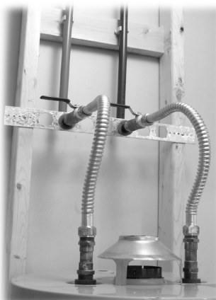
Corrugated supply lines, full-port shut-off valves, SnapClips, and stubout bracket.
