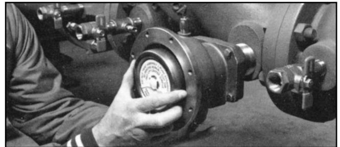
7. Replace the cover, tighten the cover bolts, and reconnect the sensing tubing. Return to service and test the assembly to ensure proper operation.
