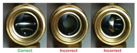
4. Once both the actuator and valve have been aligned "correctly" the actuator can be reinstalled onto the valve by sliding actuator over the valve stem until the actuator sits tight against the actuator support plate with the actuator positioned vertically as shown below.
