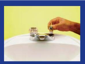
Drop in the Meter One cartridge and tighten down.
