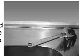
**Step A** – Drill a 1/4" pilot hole. Use a 1/2" Hole Punch and an adjustable wrench to punch the hole in the sink.
