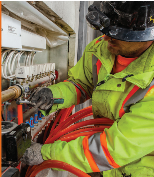
Install RadiantPERT in thin-slab systems using Watts NailTites™, or staples.
