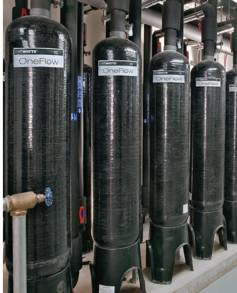
Multi-tank Parallel OneFlow® Scale Control System
