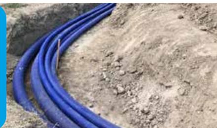
Our Microflex® pre-insulated piping system is composed of a thermal insulation around a carrier pipe and covered by a “closed chamber” protective UV-resistant outer casing. Microflex piping is suitable for use in heating, cooling, and sanitary applications allowing for reduced temperature loss and subsequent energy savings.
