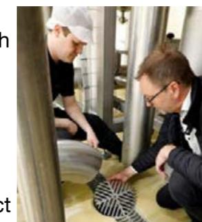
**Solution:** BLÜCHER HygienicPro® drains offer high capacity and efficient flow, are easy to clean, and help mitigate bacterial growth while limiting water volumes. They also reduce production downtime needed to maintain and clean the system. In flow comparison tests, HygienicPro drains use 96.5% less water than conventional channels. In 2022, HygienicPro customers avoided the use of 23,150 liters of water.
