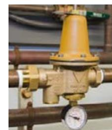
**Solution:** According to the U.S. Environmental Protection Agency, the average home can save over 11,000 gallons of water a year by reducing incoming water pressure from 80 psi to 50 psi with a pressure-reducing valve (PRV). In fact, it's estimated that Watts pressure-reducing valves avoid the use of over 19 billion gallons of water globally per year, saving water, energy, and costly wear and tear on home appliances.
