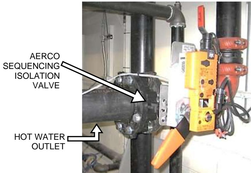
**Figure 2-20: Sequencing Isolation Valve Installed**
