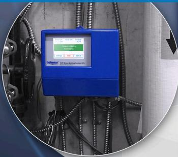
Automated flood protection systems can continuously monitor your RPZ backflow preventer.
