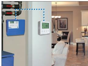
When the room temperature drops, the thermostat requests heat from the tekmar control.
