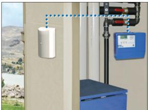
The control monitors the current outdoor temperature with an external sensor.
